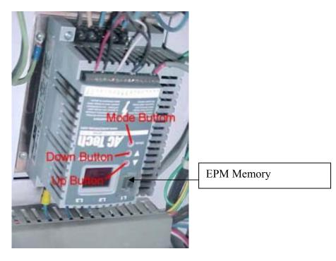
Press the **Mode Button.** The display should read "00"
